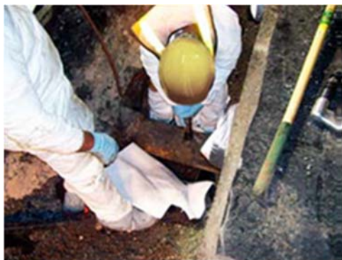
Workers tapping and draining abandoned pipelines
