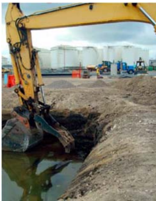
Large-scale excavation in the harbor area
